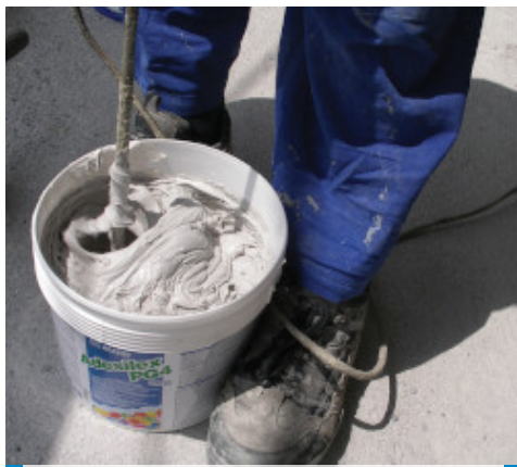
Preparing the mix
