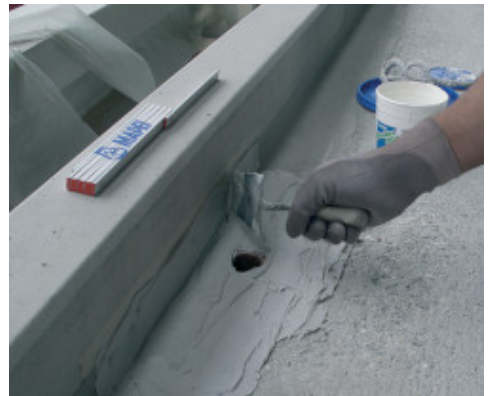
Final covering with Adesilex PG4
