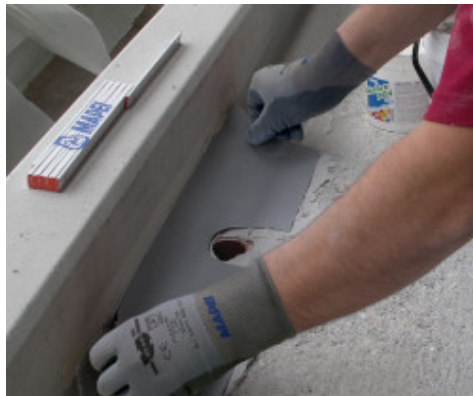
Laying flexible hyphalon brace
