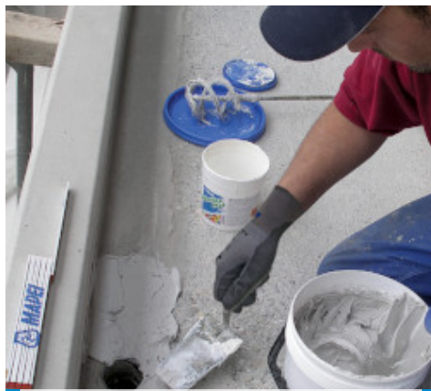
Applying Adesilex PG4 with a trowel
