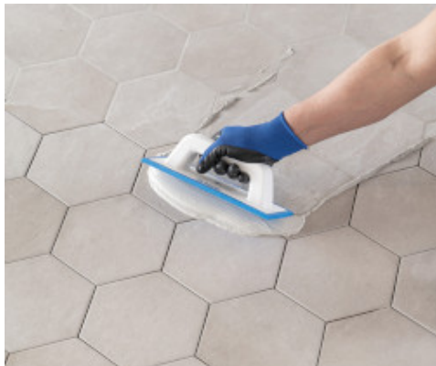
Application of Keracolor FF with MAPEI float
