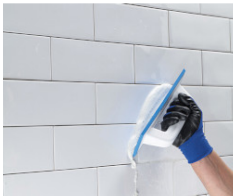
Application of Keracolor SF with MAPEI trowel
