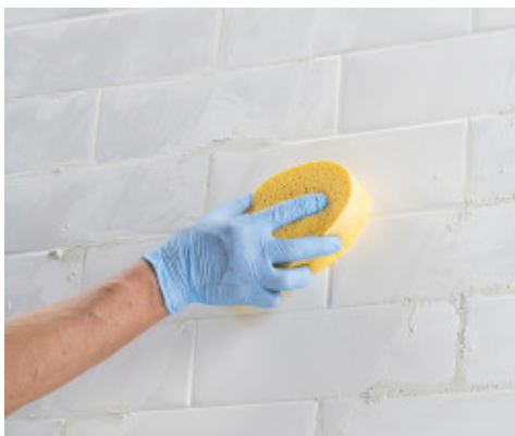
Cleaning and finishing grouts with hard cellulose sponge
